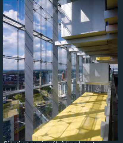
Didactic expression of building elements | Manchester Civil Justice Centre
