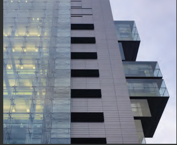
Winds intake slots for natural ventilation
